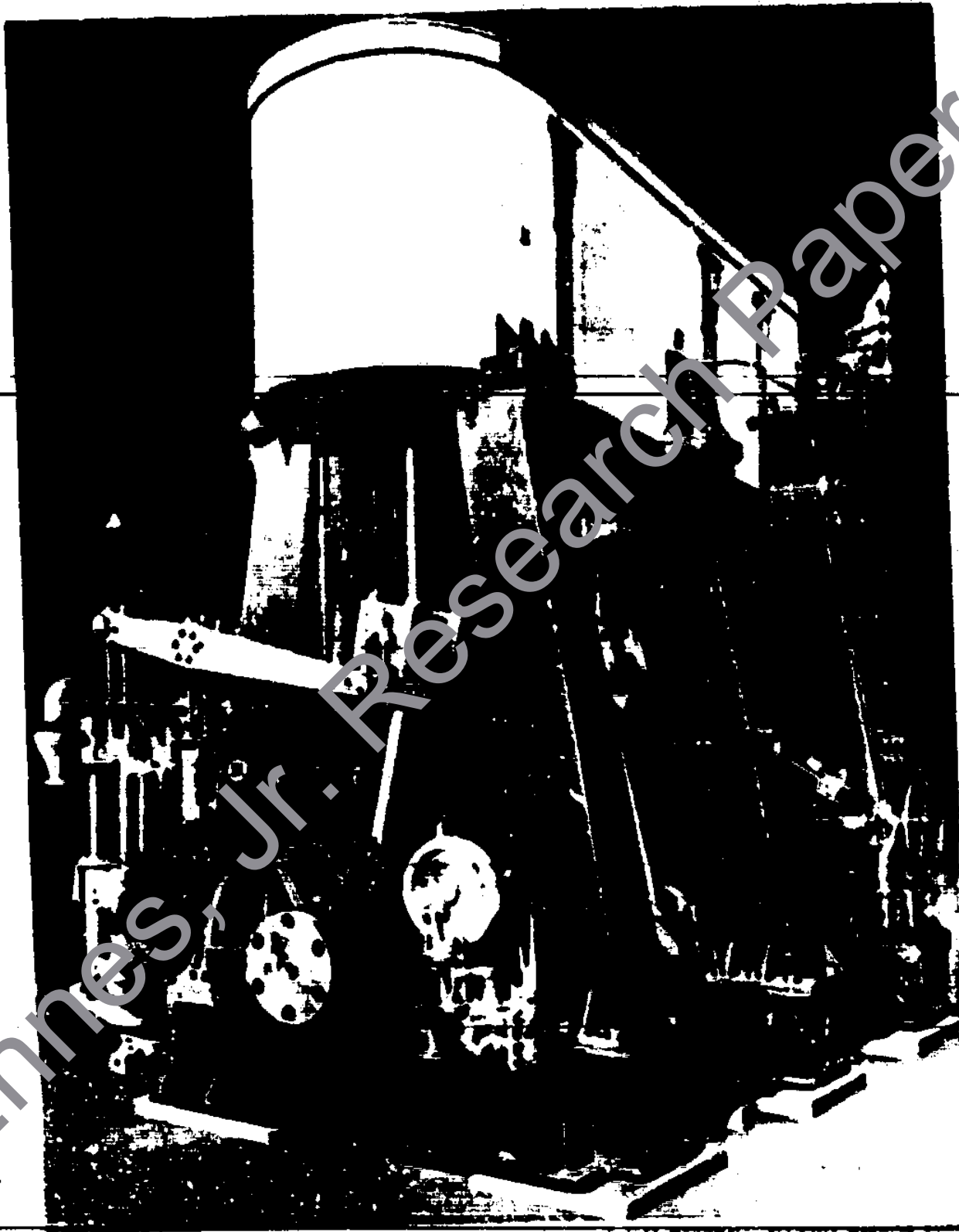
An example of the massive triple-expansion reciprocating steam engines built by the hundreds for Liberty ships in World War II. It was close to 20 feet tall.
